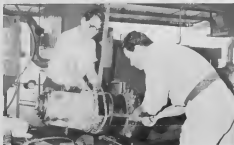
R. van der Linden and F. Croes, changing the seal of a pump.
